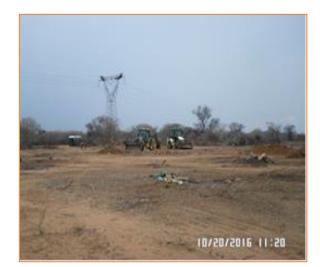
Figure 3-9: Example of clearing at tower sites
